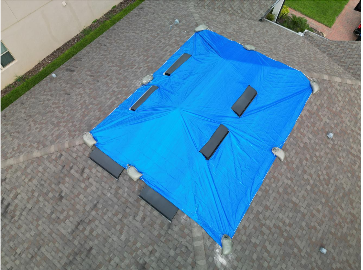
Aerial view of roof area
